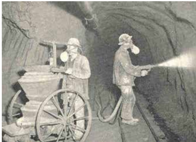
Figure 3. Lining a tunnel with gunitite using a double-chambered barrel in the 1920s (Morgan & Bernard, 2017).
