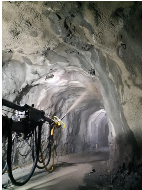
Figure 8. Tunnel under construction with projection machinery. Source: Prepared by the authors.
