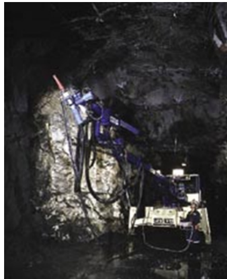
Figure 7. MEYCO Robojet Logic (Rispi, 2003).
