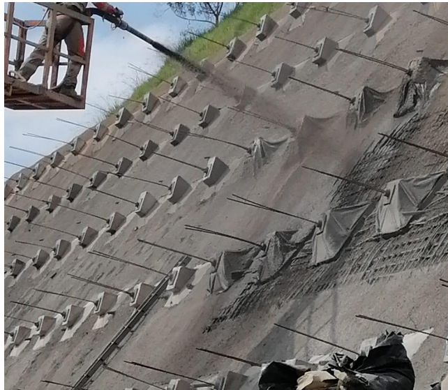
Figure 9. Slope reinforced with anchors and application of shotcrete. Source: Prepared by the authors.
